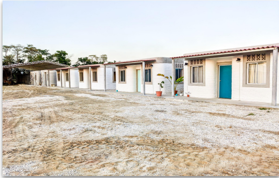
New Story: Total 6 homes printed in Tabasco, Mexico in May 2019. 500 sq. ft. structures: 2 Bdrs, 1 Bath, Kitchen, Living
