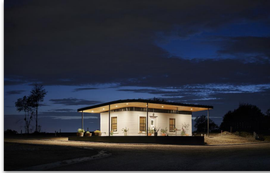
CFV Welcome Center: Printed May 2019 within 24 hours. 500 sq. ft. structure: 1Bdr, Office, Kitchen, Living
