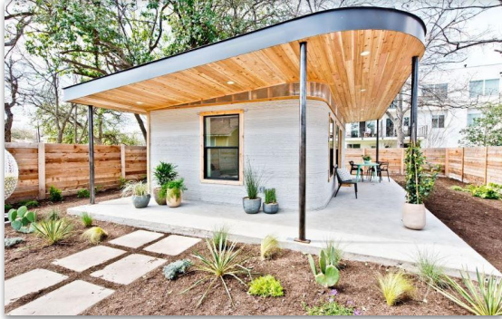
The Chicon House: Printed March 2018 within 48 hours. 350 sq. ft. structure: 2 Bdrs, 1 Bath, Kitchen
