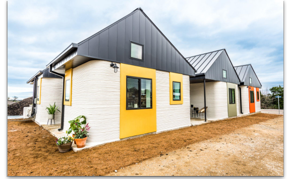
Community First Village (CFV): Total 6 homes printed in March 2020. 400 sq. ft. structures: 1 Bdr, Kitchen, Living
