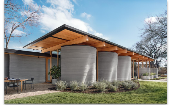
House Zero: Printed in Winter 2021 within 10 days. 2,000 sq. ft. structure: 3 Bdrs, 2.5 Bath with a 350 sq. ft. ADU
