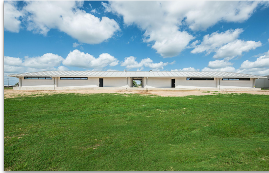
Camp Swift Barracks: Printed in August 2021, 3,800 sq. ft. structure set to house 72 soldiers
